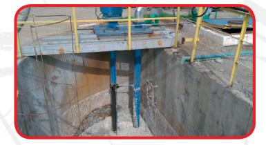
Vertical pump with vortex impeller. 6 meters length. The vertical immersible sump pump is installed in external sump that collects wastewater from paper pulp process. All the intermediate bearing bushes, four in this execution, are lubricated by an external source: bushes are always in contact with clean liquid.
